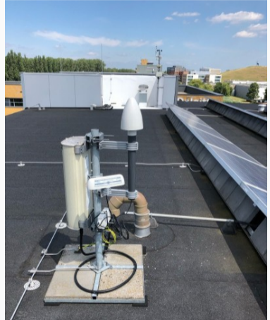
Figure 1: GPS/Galileo and DCF77 antennas on SIDN's roof
